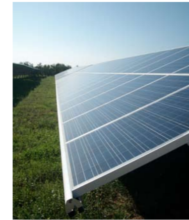
Q-Cells, 6MW in 6 solar parks
